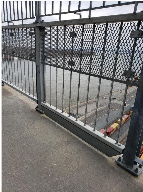
Figure 37 : Kick-back plate in the lower part of the guardrails
