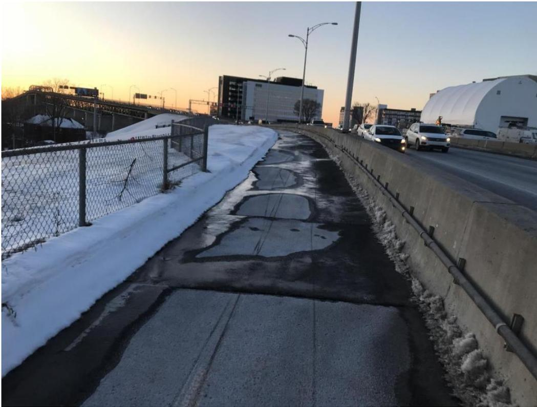
Figure 19 : Slush edge leaving water puddles on the multipurpose path that are conducive to freezing
