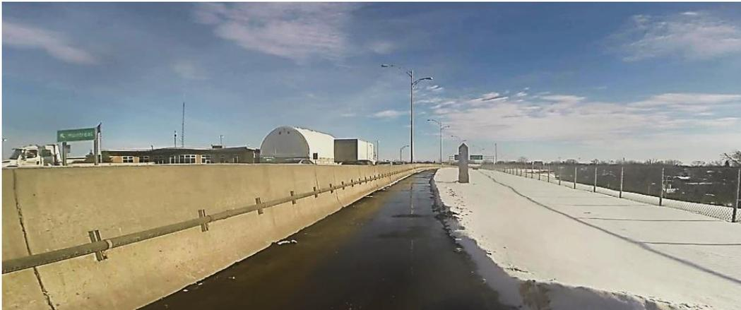
Figure 13 : Wet and undrained surface at Section 2 of the Jacques Cartier Bridge
