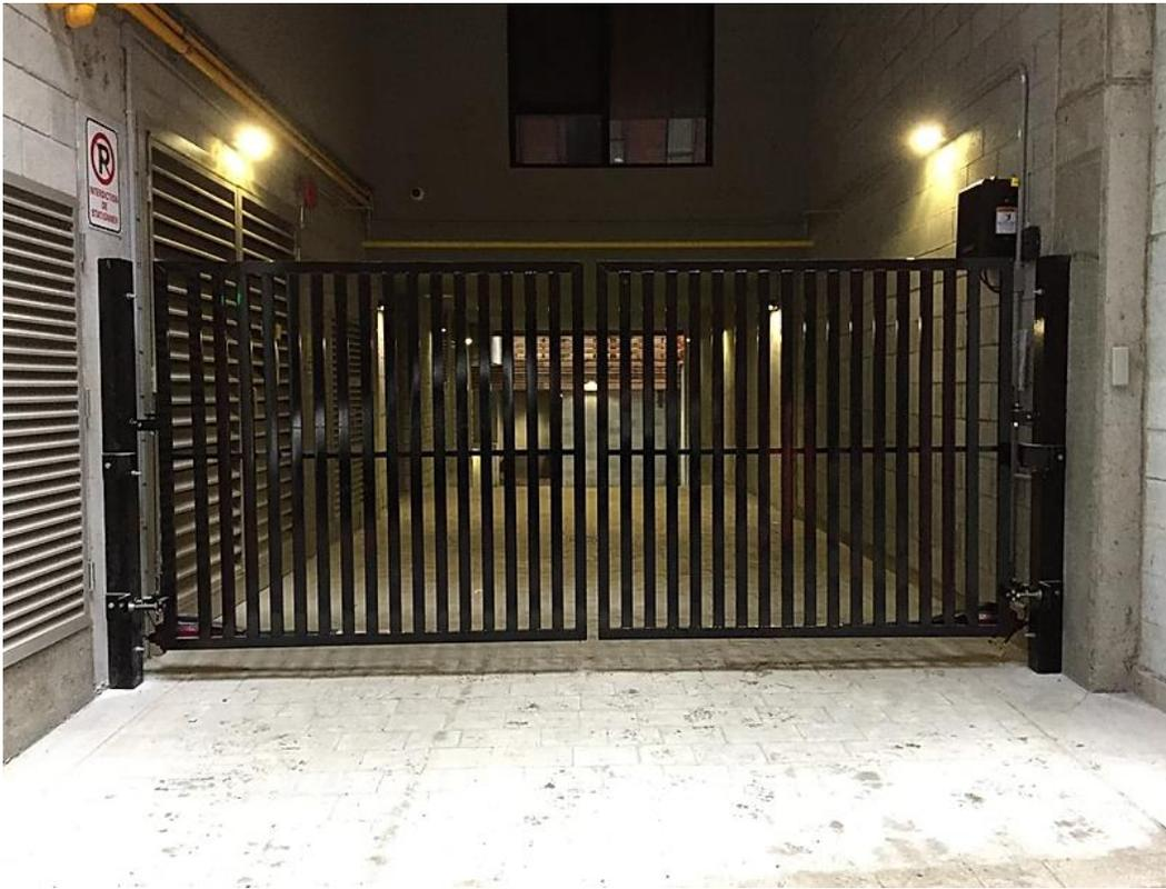
Figure 44 : Example of an automated barrier [MastergatePlus]
