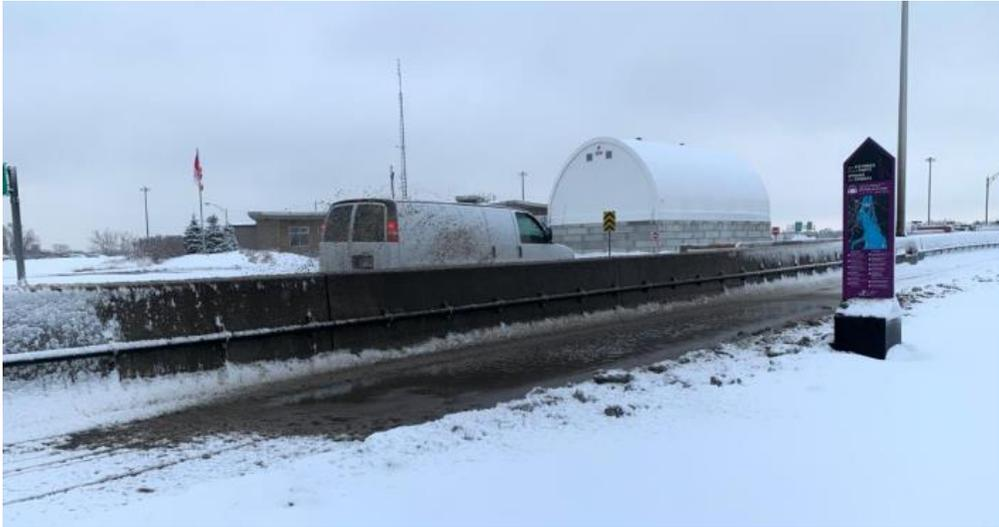
Figure 17 : Splashes of dirty water from the road on the multipurpose path
