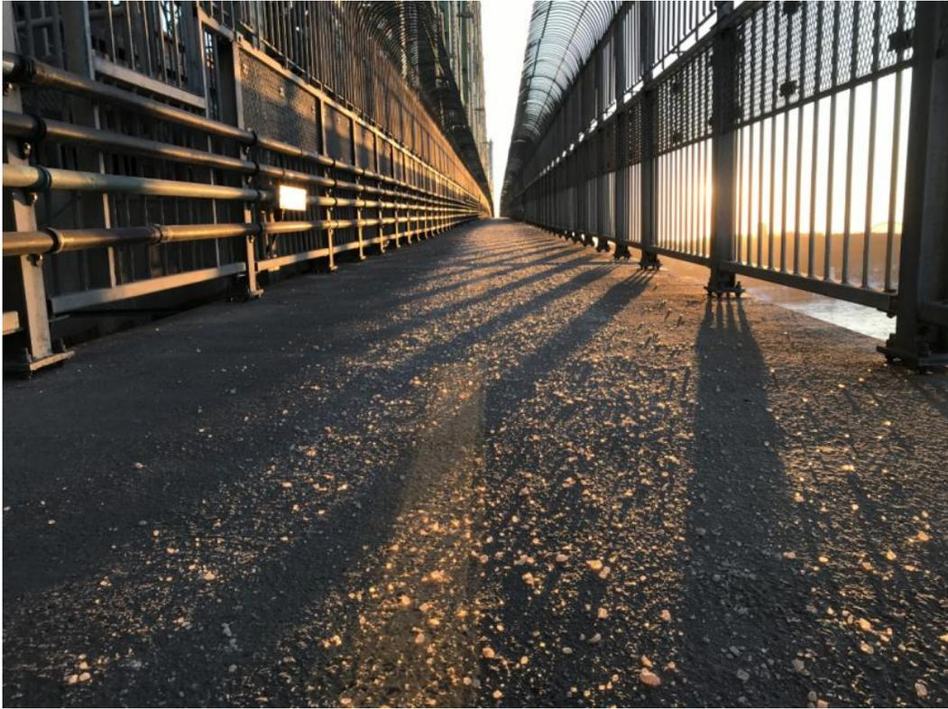
Figure 18 : A large amount of de-icing products spread on the multipurpose path
