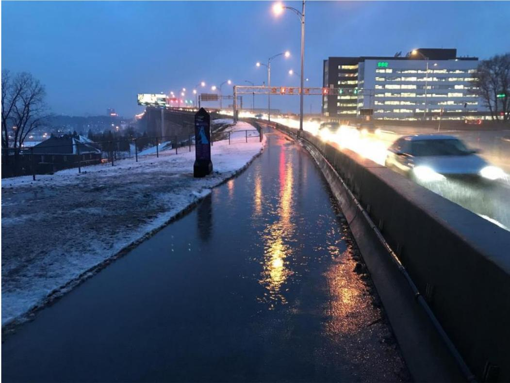
Figure 20 : Puddle in Section 1 of the bridge
