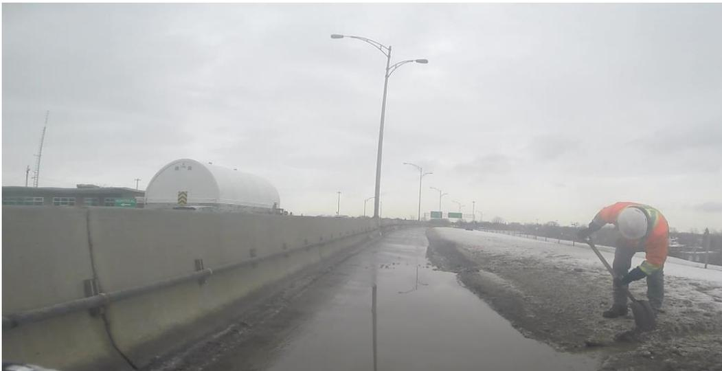
Figure 21 : A worker creates a path to evacuate water from the path
