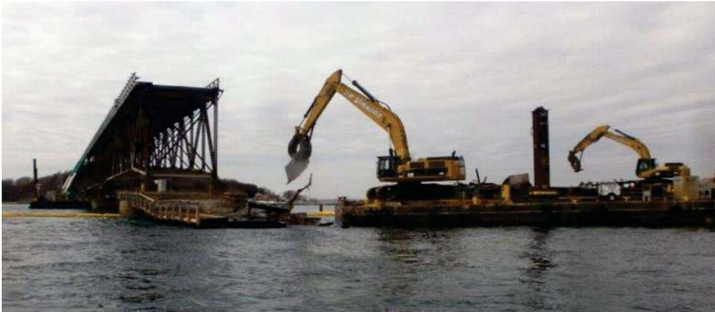
Figure 37 – Standard barge method used for the deconstruction of the Long Island Bridge in Boston Harbour (source: Walsh Construction 2016)
