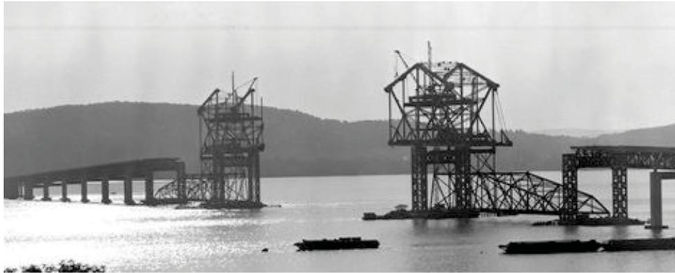
Figure 50 – Tappan Zee Bridge Construction using Balanced Cantilevers courtesy of Westchester County Historical Society)
