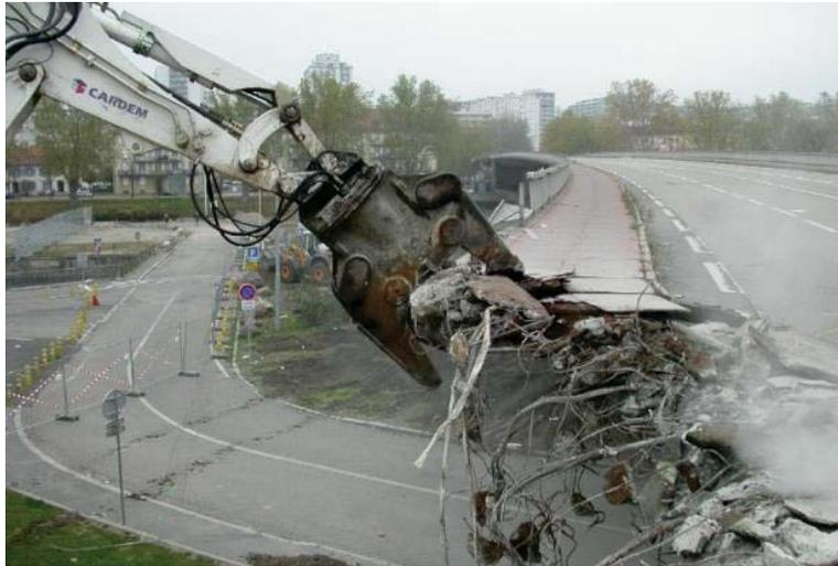
Figure 39 – Deconstruction of bridge deck using a concrete crusher with shear jaws
