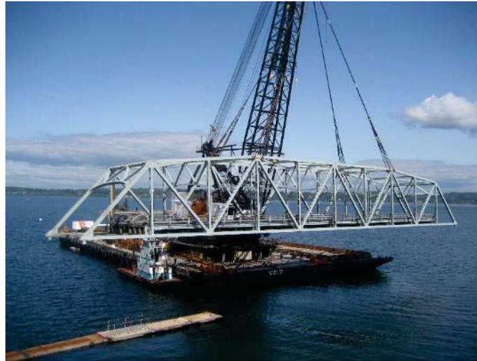
Figure 56 – Hood Canal Bridge Removal
