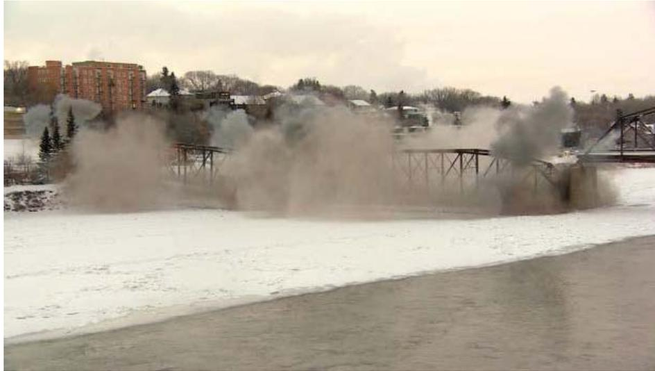
Figure 68 – Deconstruction of Saskatoon Traffic Bridge using an ice bridge (source: Radio-Canada 2016)
