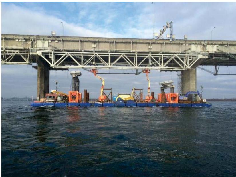
Figure 114 – Sectional Barges used to Install the trusses of the Champlain Bridge
