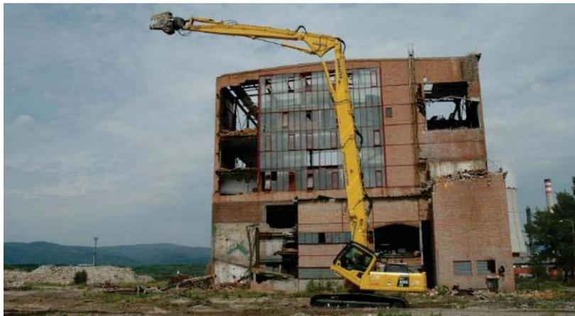
Figure 38 – Concrete crusher with shear jaws mounted on a telescopic-arm excavator (source: Marubeni-Komatsu, 2016)
