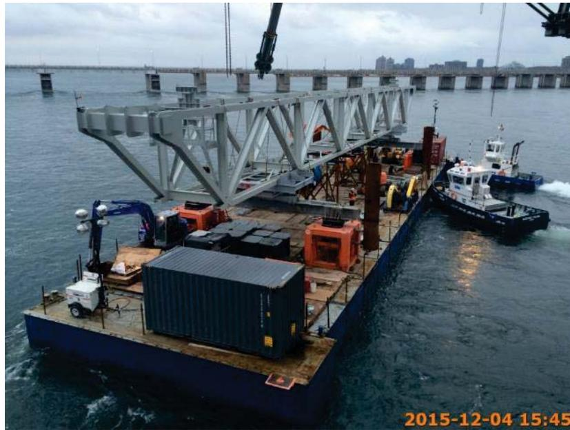
Figure 115 – Sectional Barges Used to Install the trusses of the Champlain Bridge
