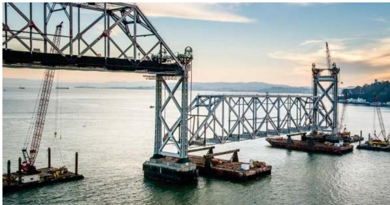
Figure 54 – San Francisco Oakland Bay Bridge – 504' Span Dismantling
