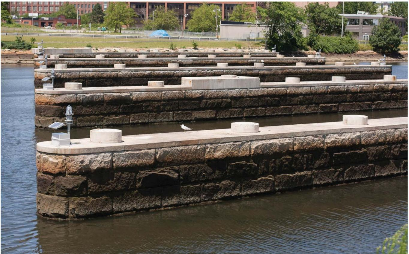
Figure 12 – Detailed view of existing pillars that will be used as foundation for the new pedestrian bridge. Source: City of Providence, 2014
