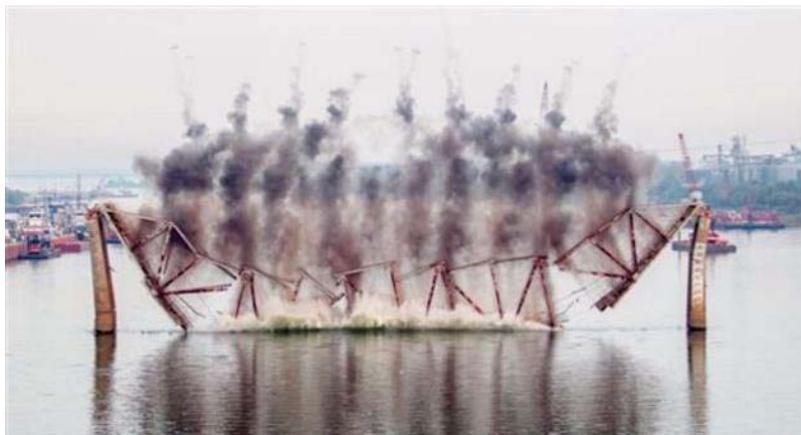
Figure 47 – Explosive Deconstruction of Old Ledbetter Bridge (source: [www.courierpress.com](http://www.courierpress.com))
