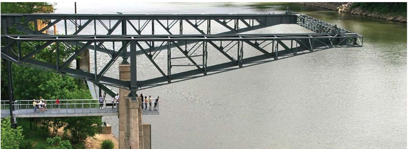
Figure 2 – Footbridge under the old retractable bridge. Source: Landezine, 2013
