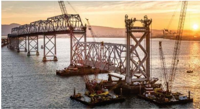
Figure 52 – San Francisco Oakland Bay Bridge – 504' Span Dismantling (source: courtesy of Foothills Bridge Co (Photo by Sam Burbank))
