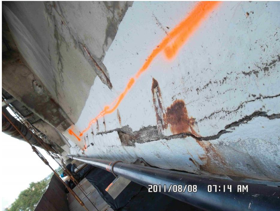
Fig. 11.2: Condition of bottom flange of Girder P7 in span 10E-11E in August 2011.
