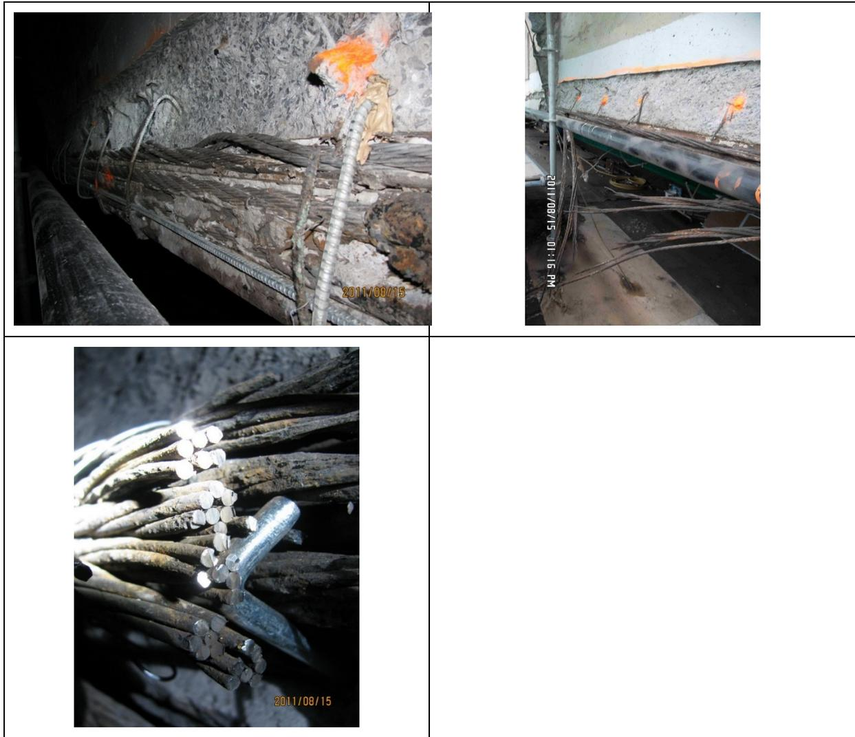
Fig. 11.5: Concrete removal and condition of GTM strands during repair of bottom flange of Girder P7 in span 10E-11E in August 2011.
