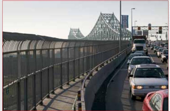
The Bridge is in relatively good condition however the bridge is now over 80 years old and certain elements will require repairs in the next few years, notably repairs to the piers, replacement of bearings, repairs to certain steel components and renewal of the roadway pavement and painting.
