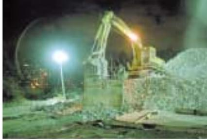
Demolition of old slabs from bridge, to be recycled as aggregate
