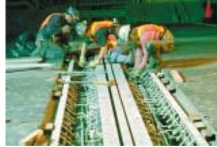
Adjustment of a section of the three-module expansion joint
