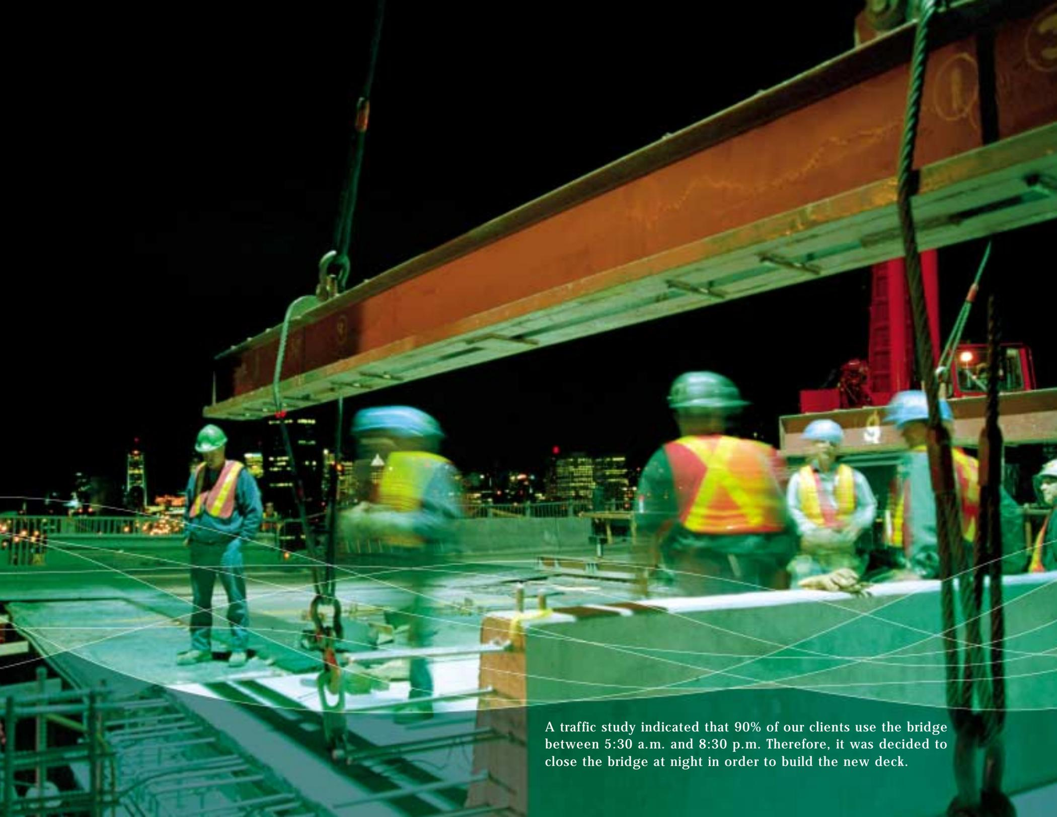
A traffic study indicated that 90% of our clients use the bridge between 5:30 a.m. and 8:30 p.m. Therefore, it was decided to close the bridge at night in order to build the new deck.
