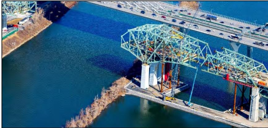
Deconstruction of the steel structure of the Champlain Bridge
